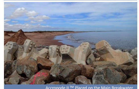
Accropode II™ Placed on the Main Breakwater
