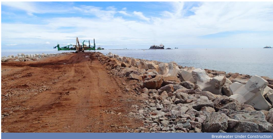
Breakwater Under Construction
