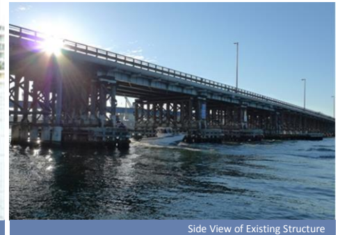
Side View of Existing Structure
