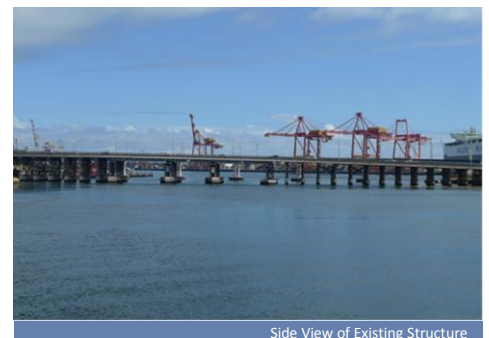
Side View of Existing Structure
