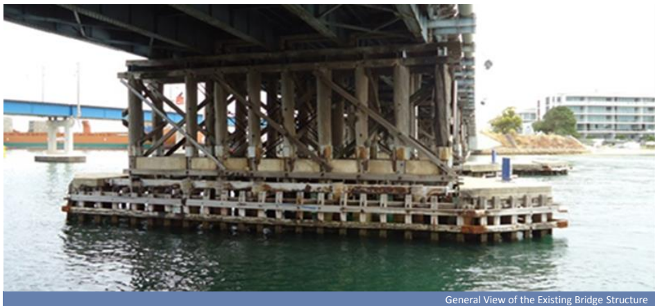
General View of the Existing Bridge Structure
